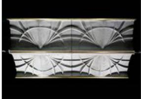
"although optimization algorithms can significantly reduce the amount of concrete used on complex buildings, the construction industry remains limited by the available fabrication technologies. to tackle this problem, digital building technologies, ETH zürich has proposed an automated solution that combines the fabrication speed of concrete 3D printing with the geometric precision of reusable 3D printed formwork."
