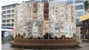
"While materials ranging from concrete to insulation are wrecking our environment, the Growing Pavilion is made entirely from materials that grew on this planet."
