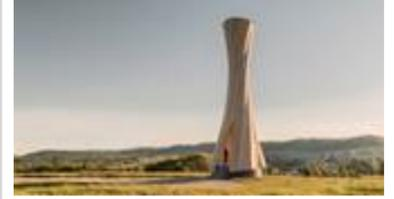
"University of Stuttgart engineers have harnessed the natural shrinking process of wood as it loses moisture to create this world-first self-twisted tower in Germany."
