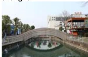
"The fabrication of the bridge comprises a 3D printing concrete system independently developed by Professor Xu Weiguo's team. The concrete components of this bridge had been entirely printed with two robotic arm 3D printing systems over the course of 450 hours."
