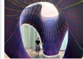
"With just the press of a button, ETH researchers knit a textile that serves as the primary shaping element for curved concrete shells. Now they have used the new technology to create a five-tonne concrete structure for an exhibition in Mexico City."
