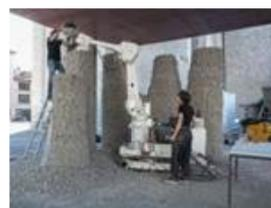
"No cement. No nails. No screws. This robot arm needs just two things to build structures: gravel, and a really, really long string."
