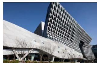
"Aramid, the material Morphosis chose for the interconnected sunshade system, is a reinforced fibre manufactured by Kolon that has five times the tensile strength of iron. It is used in everything from bullet-proof vests to aircraft parts."
