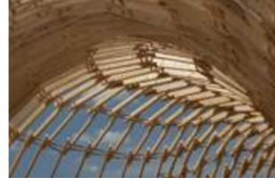
"The four-metre tall construction was inaugurated in June and was the handiwork of 17 architecture students at the Swiss Federal Institute of Technology in Zurich (ETHZ). The structure is made completely of timber and is held together by 2,700 cylindrical wooden pegs called dowels."
