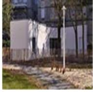
"The house took a little more than 2 days to print ... The construction of the entire house cost around £176,000. This means that the cost of construction done by 3D printing is 20% cheaper than using conventional construction techniques."
