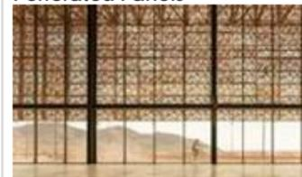
In order to establish a new Morocco airport which embraces natural light and ventilation, architects adorned the facade of the building with perforated panels.
