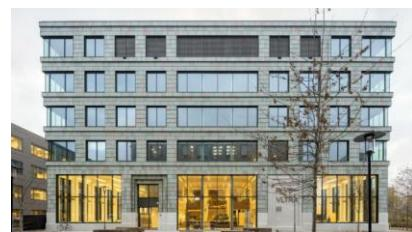
"Dutch manufacturer Pretty Plastic has created the facade for Plus Ultra III, the first timber laboratory building in the Netherlands, using tiles made from recycled post-consumer plastic waste."
